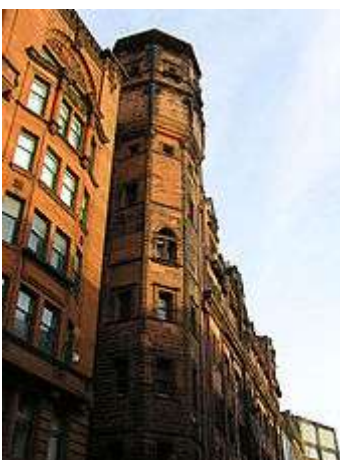
"The Lighthouse", Charles Mackintosh's Glasgow Herald building
